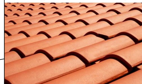
Roof covering and different color flat facade plates
